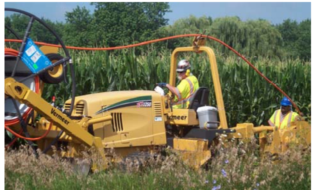
Workers plow south of the Sublette site to prepare the path.
