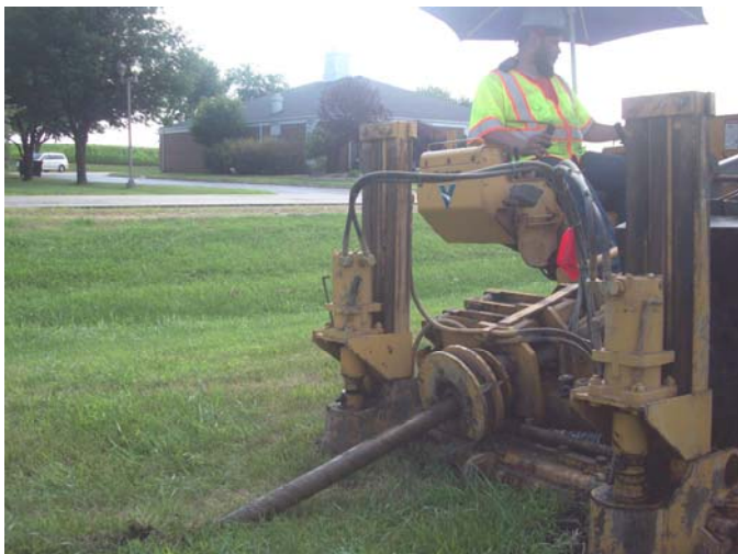
The cable bores underground to workers waiting several hundred feet away.
